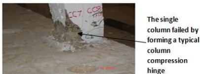
**Fig. 12(g): Crack due compression in column C2 and spalling of concrete**
