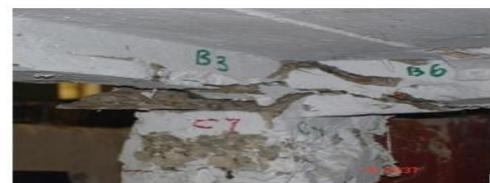
**Fig. 12(c): Crack in C<sub>7</sub>-B<sub>3</sub>-B<sub>6</sub> joint (Column - Beam Interface Crack) and spalling of concrete at beam-column junction**
