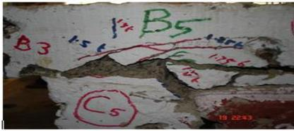
**Fig. 12(d): Crack in C5-B3-B5 joint (Column-Beam Interface Crack) and spalling of concrete in beam-column junction**
